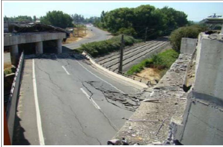
FIGURA 3.2. Colapso PS Hospital, (FHWA, 2011).
