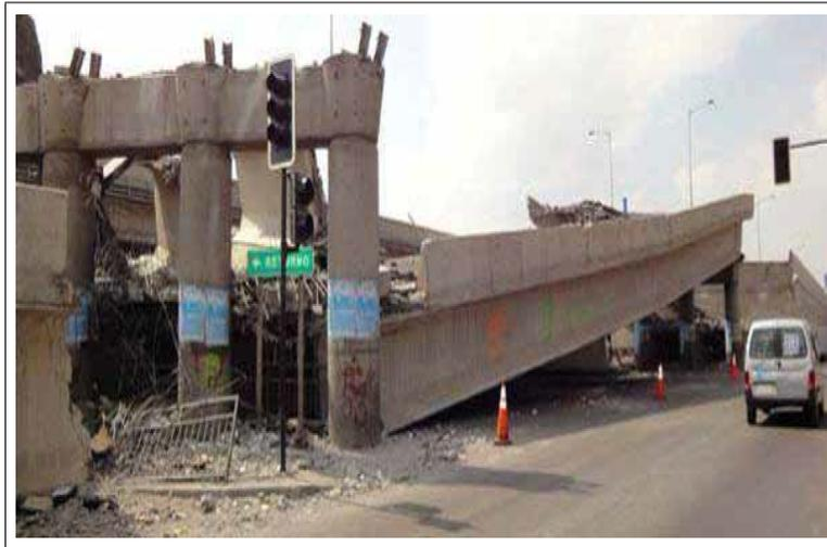
FIGURA 3.3. Colapso PS Lo Echevers, (FHWA, 2011).
