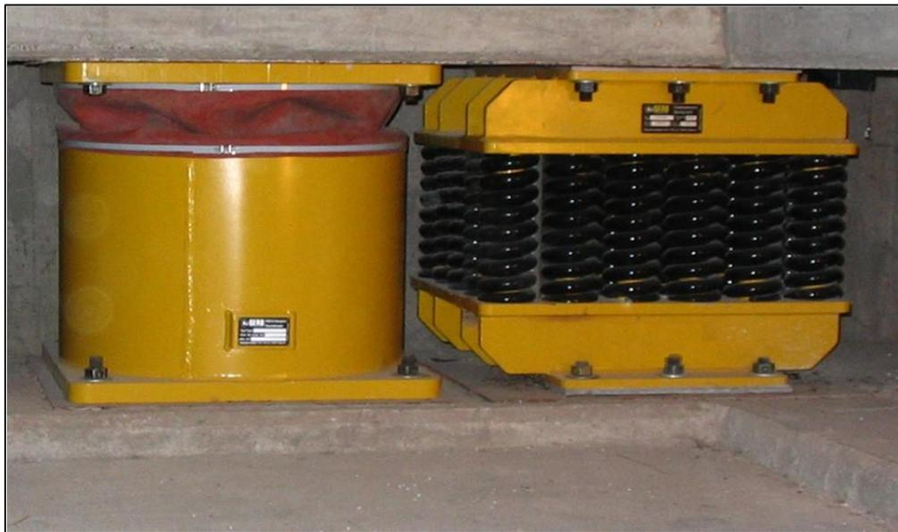
Figure 1.2. Typical Base Control System below apartment building (Nawrotzki et al, 2019).
