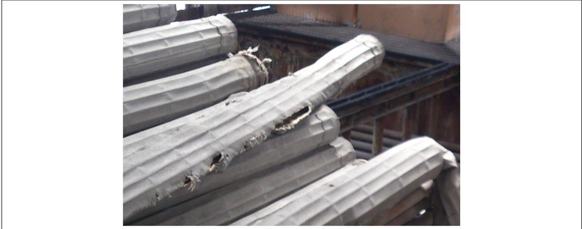
Figure 1.5. Damaged fabric filters for replacement (Photo by G. Lara)
